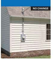
The electric line that serves the neighborhood would be placed underground, but the service line providing power to the house would remain overhead.
