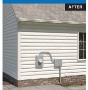
A stainless steel "horizontal box" adapter is used in areas susceptible to sea salt. It can be installed utilizing entrance cable to connect the meter base to the adapter.
