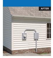
A "vertical box" adapter can be installed utilizing entrance cable to connect the meter base to the adapter.
