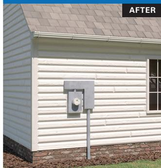
An "ELL" adapter can be installed near the current meter base.
