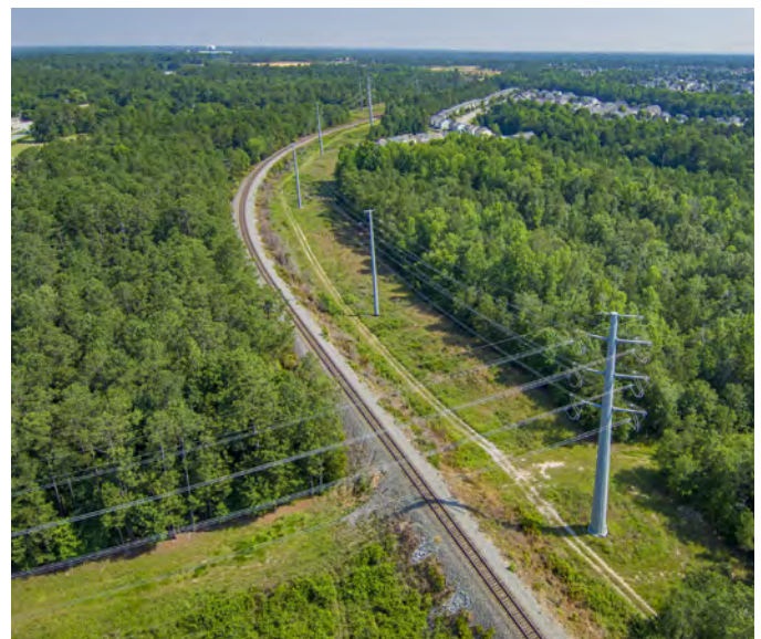
VCS1 - Killian 230KV and Blythewood Switching Station – Killian 115KV Transmission Lines
