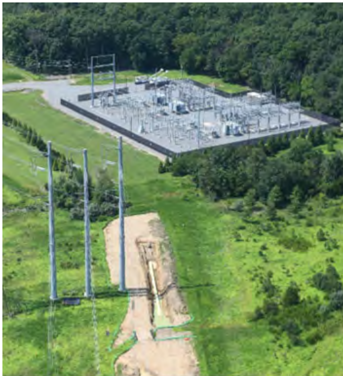
Double Circuit 3-Pole Double Deadend
