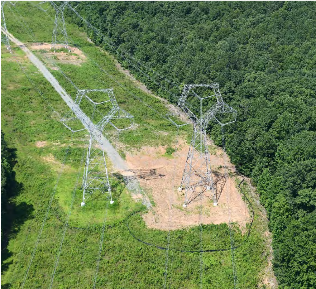
93MA Running Angle Tower (534/568)
