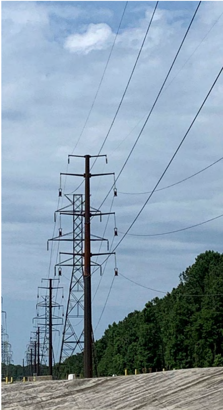
Typical Double Circuit Suspension Monopole Structure
