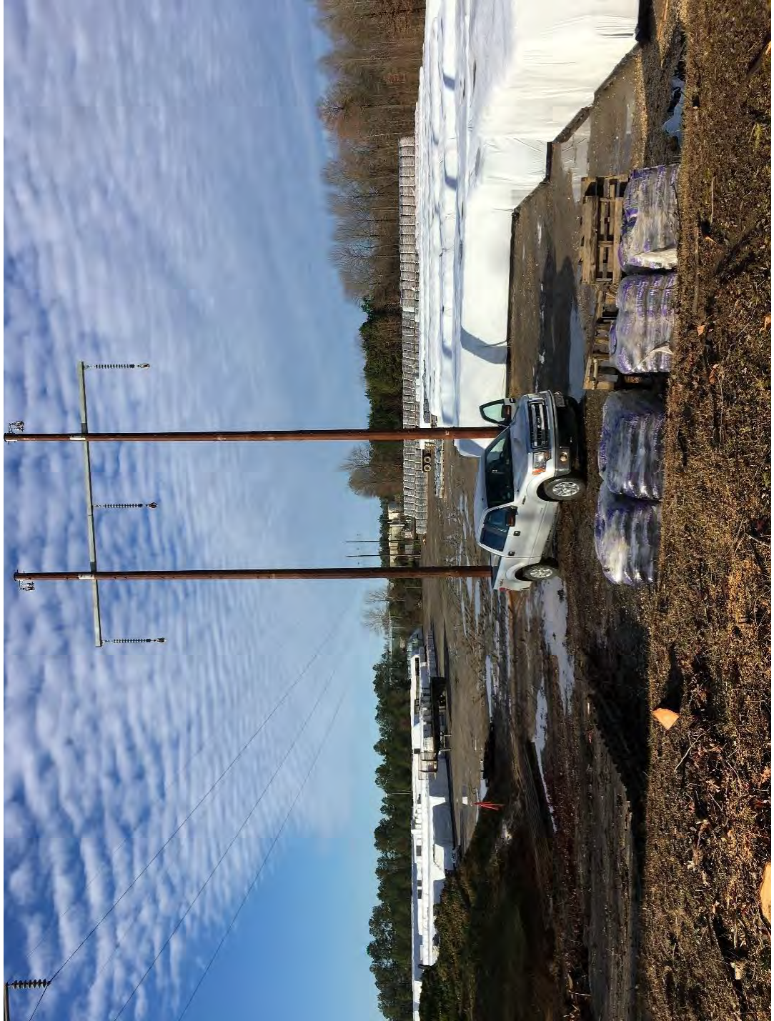
Typical Single Circuit Suspension H-Frame Structure
