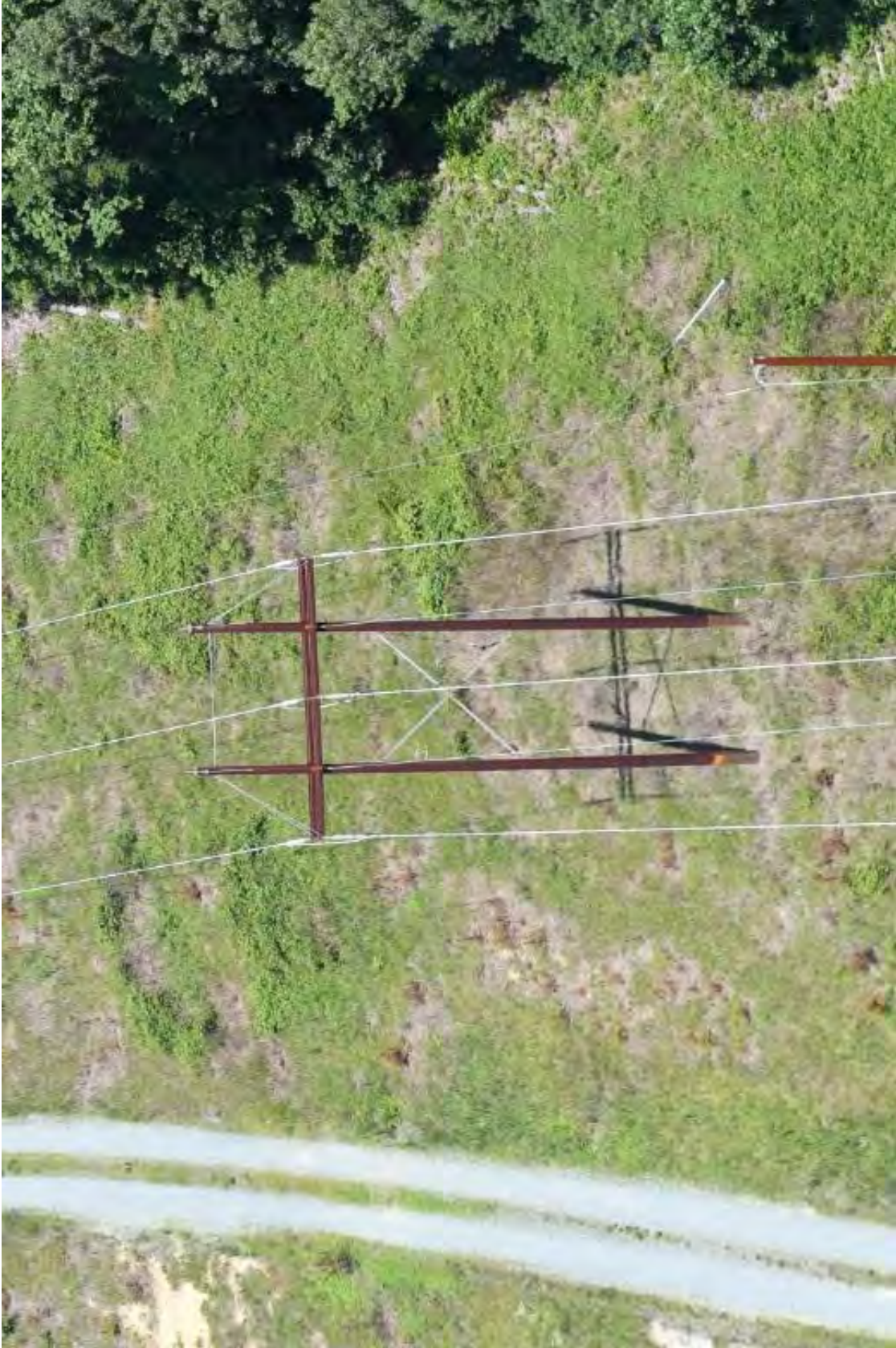
Typical Single Circuit Deadend H-Frame Structure
