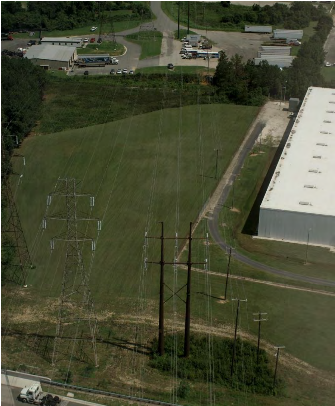
Typical Double Circuit H-Frame Structure
