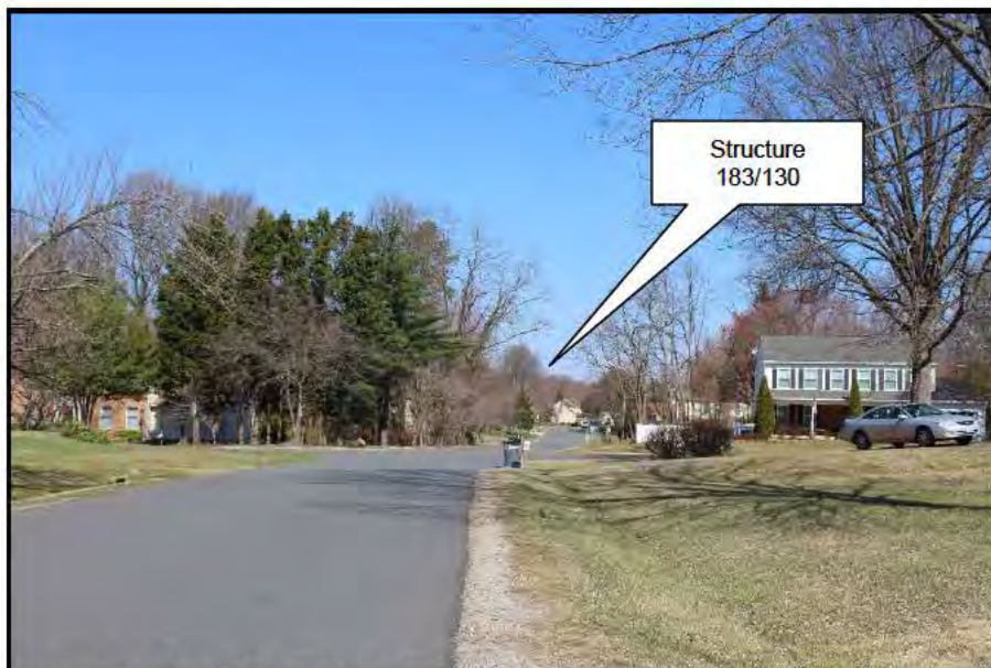
Figure 6 View from Bel Air (DHR #076-0001), Looking North from Location 3. The Existing Transmission Line is Visible.
