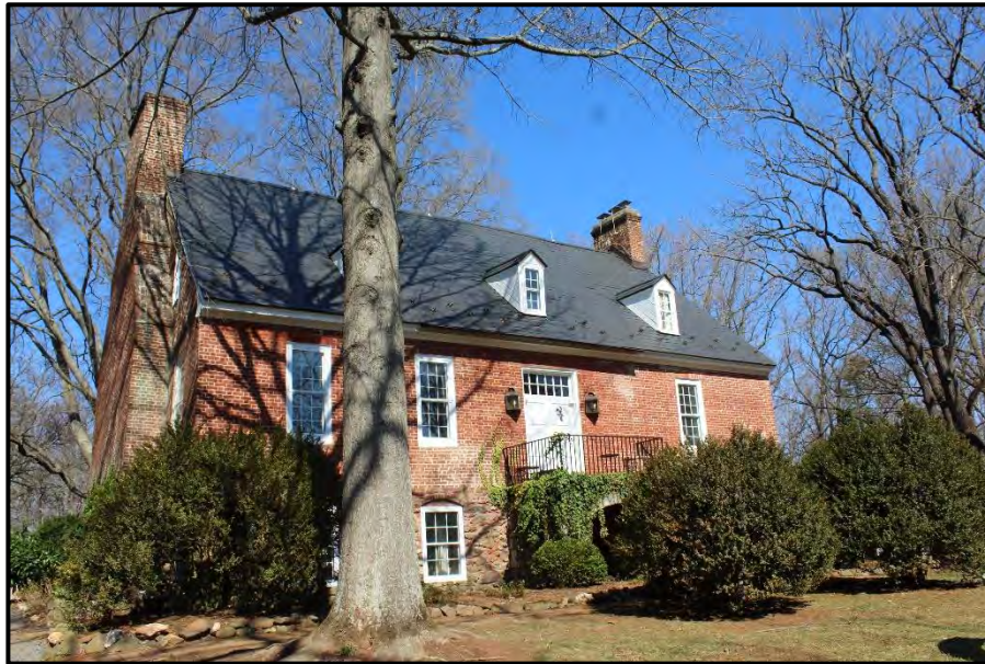
Figure 2 View of Bel Air (DHR #076-0001), Looking North.
