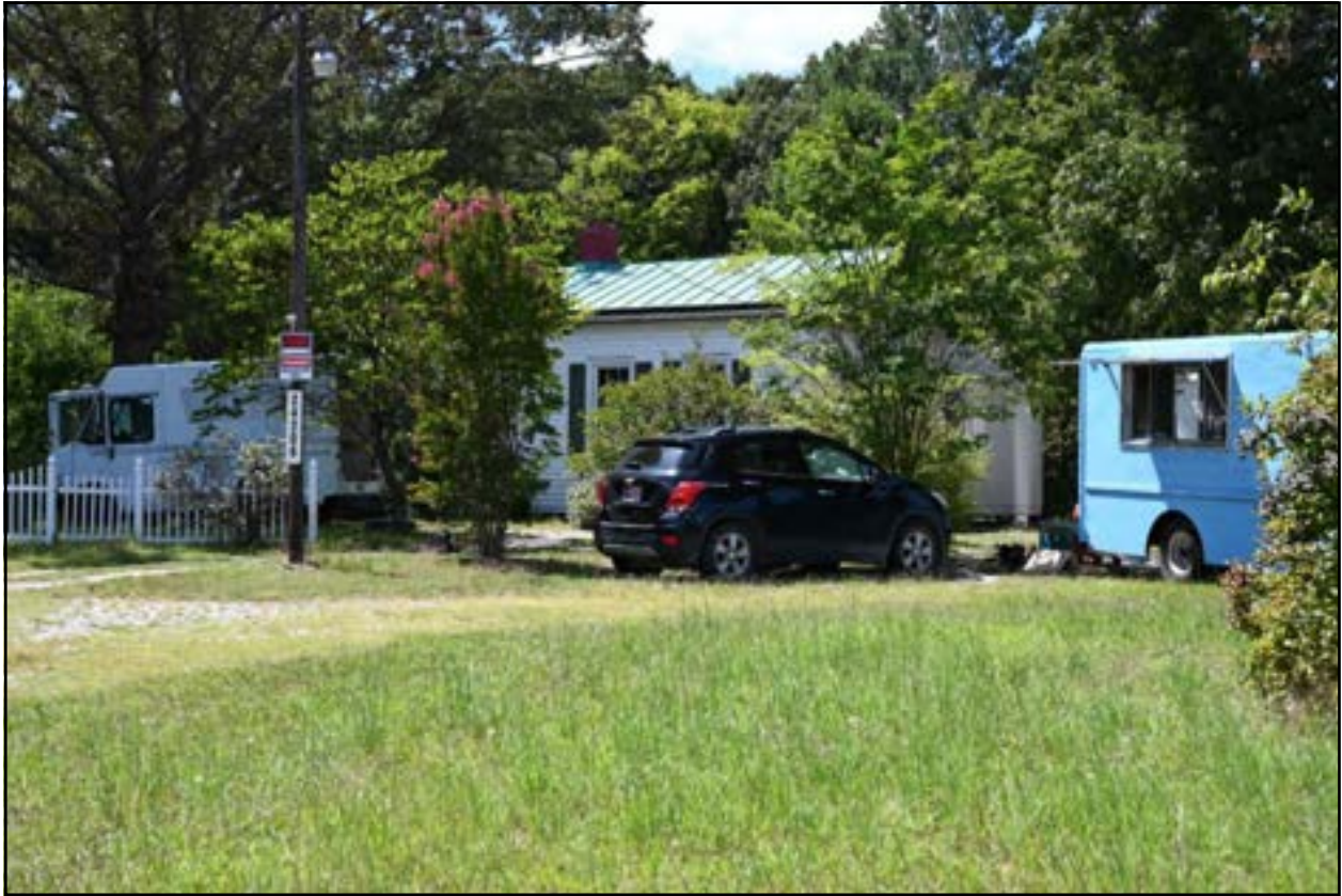
Figure 1. 016-5097, Rosenwald School, View to the Southwest.
