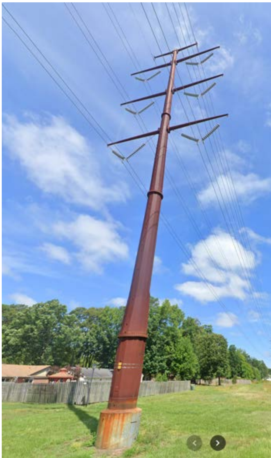
Double Circuit Engineered Monopole Suspension Structure (V-String)
