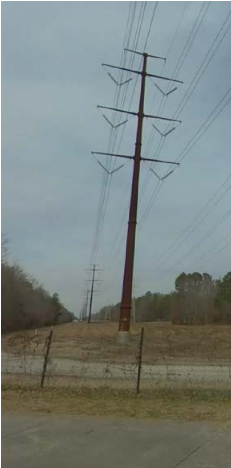
Double Circuit Engineered Monopole Suspension Structure (V-String)
