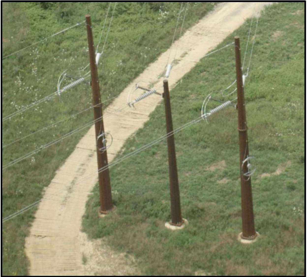
230kV SC 3 Pole Heavy Angle DDE
