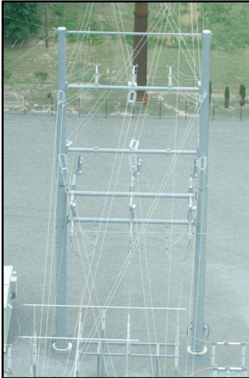
Proposed Double Circuit Backbone
