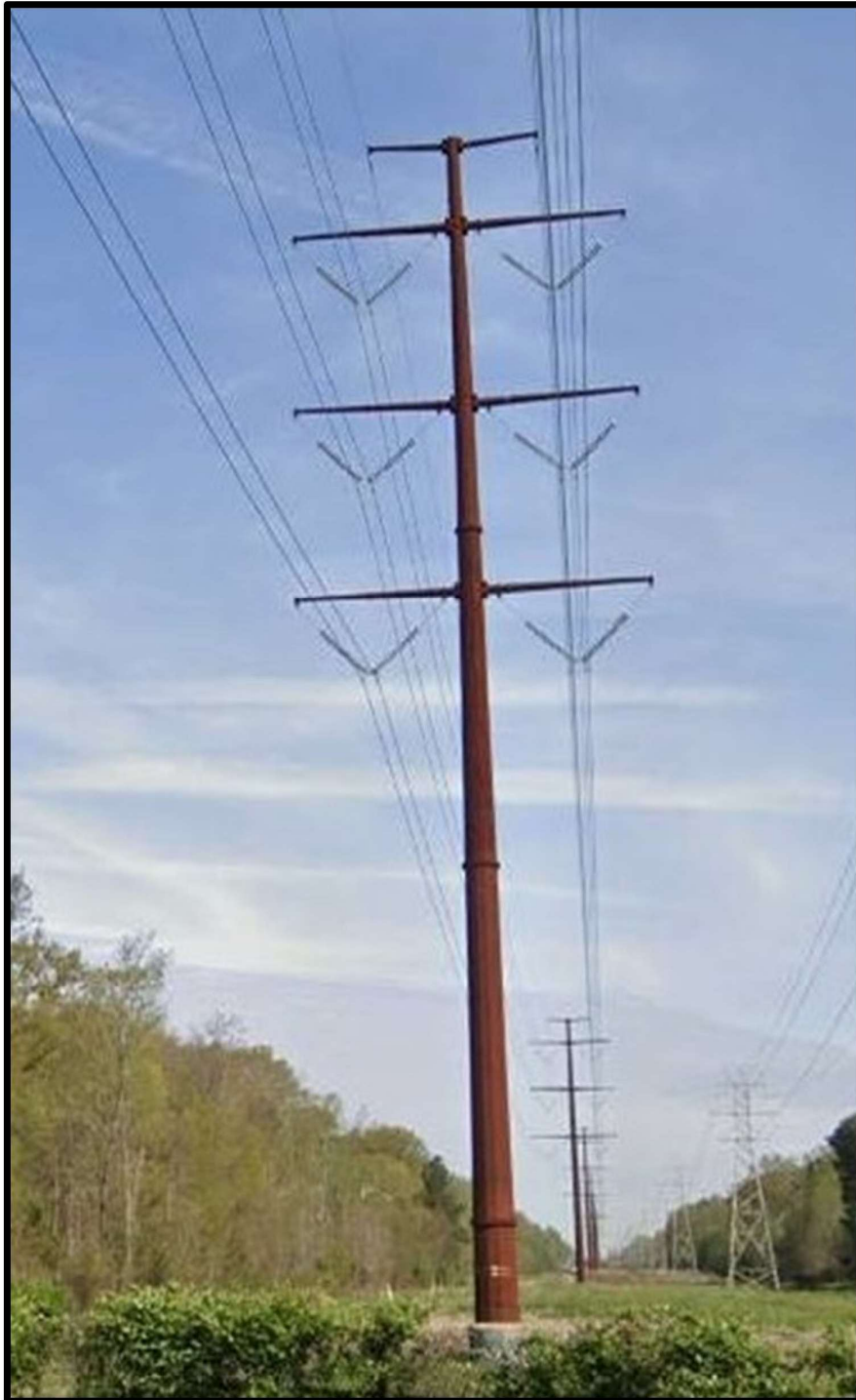
Proposed Double Circuit Tangent V String Suspension
