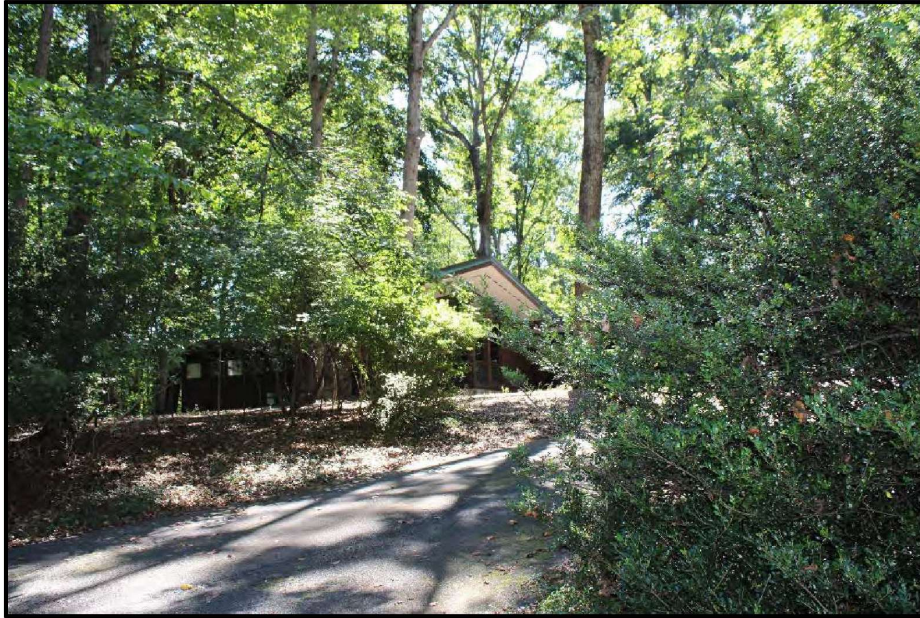
Figure 42. Thomas and Alena Hammond House (DHR #104-5995; PL 44), Looking Southeast.
