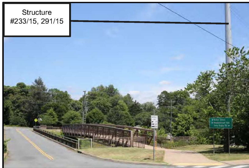
Figure 92. View from Meadowbrook Hills Historic District (DHR #104-5394; PL 52) at ROW on St. Anne's Road, Looking Northeast. Existing Transmission Line is Visible.
