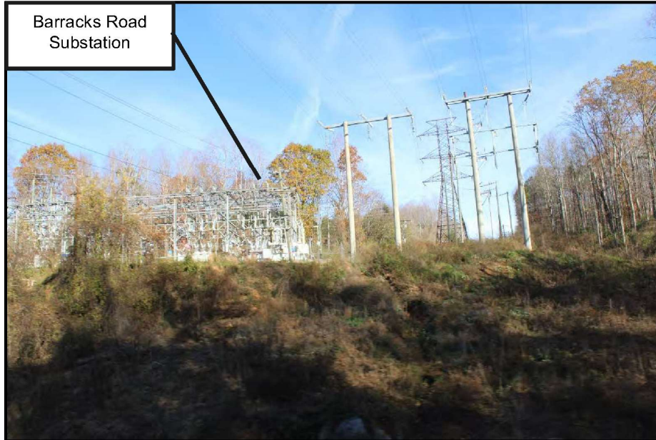
Figure 113. View from Farmington Historic District (DHR #002-5153; PL 27) Looking East. The Existing Transmission Line and Substation is Visible.
