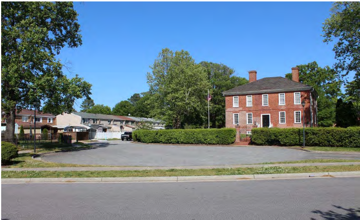
Figure 5-3: Photo location 2- General view of Pembroke Manor setting, facing northeast.
