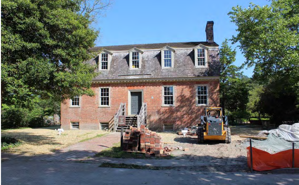
Figure 5-16: Photo location 1- View of Francis Land House, front façade, facing southeast.
