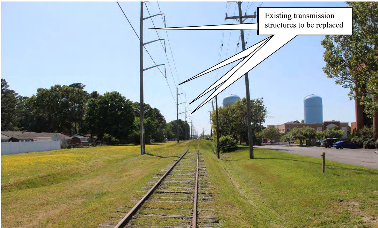
Figure 5-28: Photo location 2- View of corridor and existing transmission line from Kellam Road crossing, facing west.
