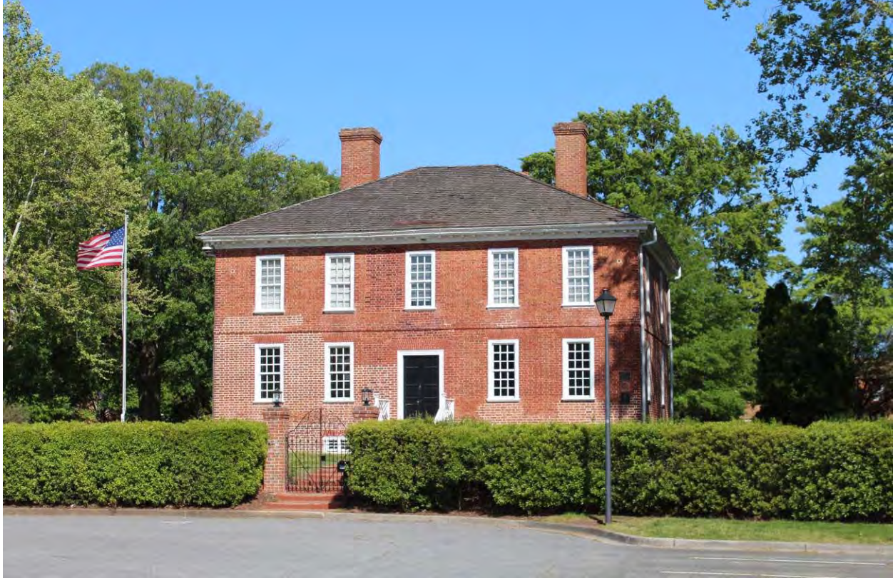
Figure 5-2: Photo location 1- View of Pembroke Manor, front façade, facing northeast.
