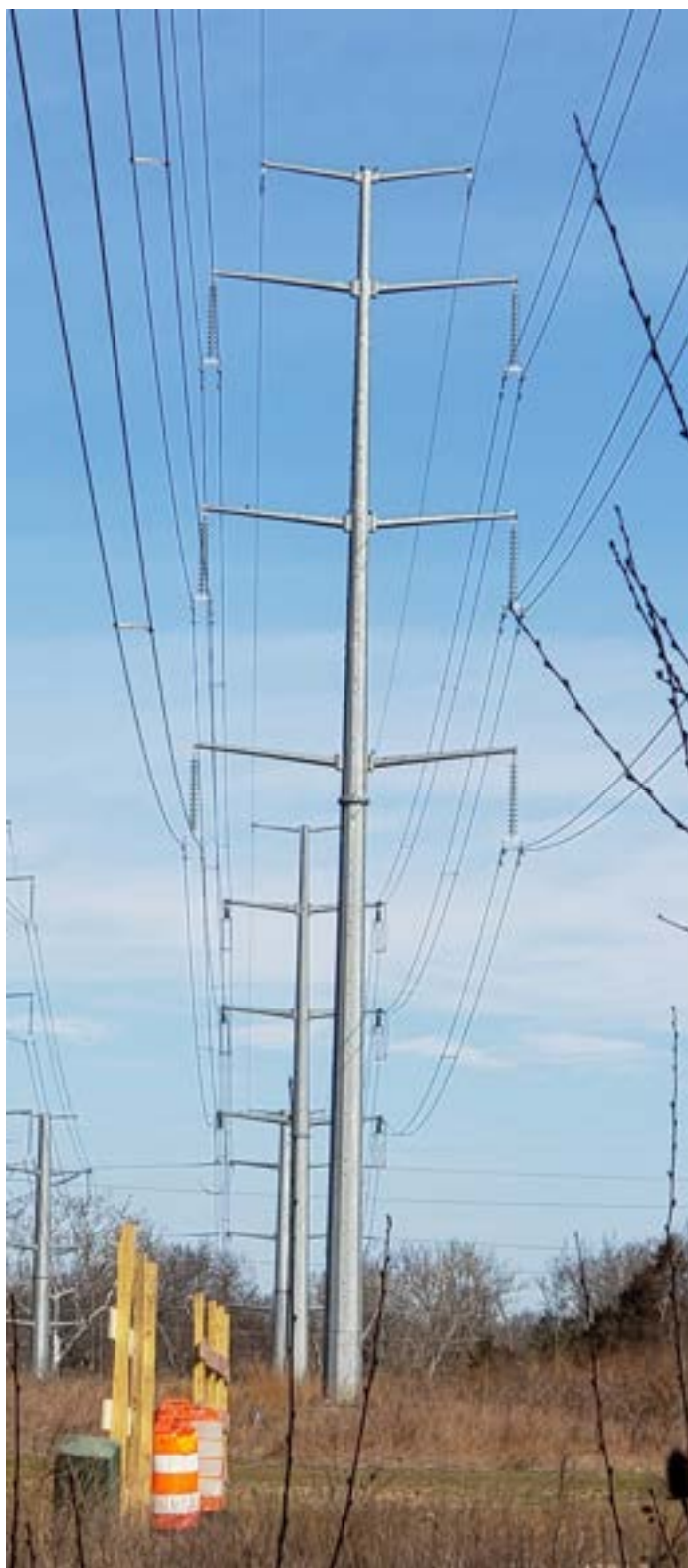
Existing Structure Type: 230kV Double Circuit Steel Monopole (TAN)
