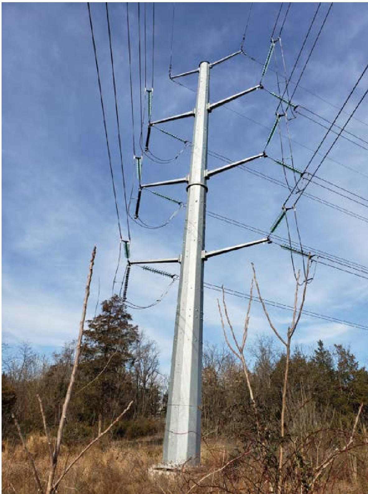
Proposed Structure Type: 230kV Double Circuit Steel Monopole (DDE)
