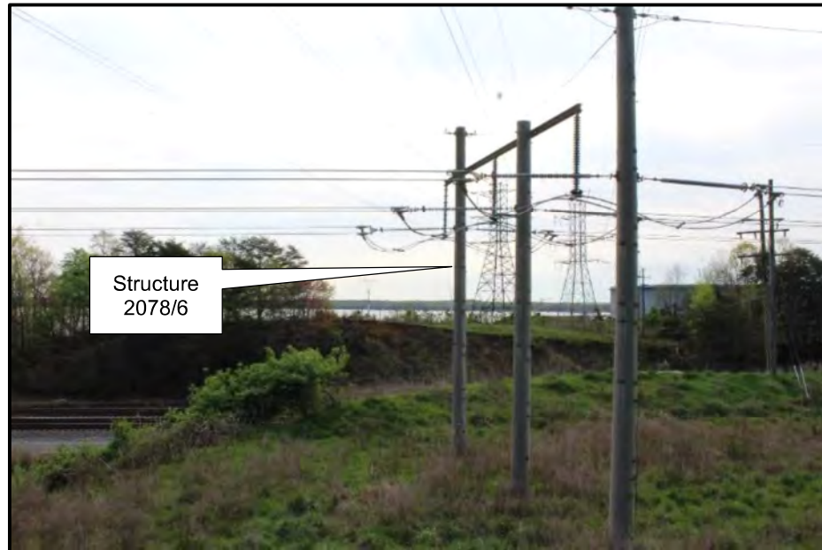
Figure 9 View from Richmond, Fredericksburg & Potomac Railroad (VDHR #076-0301), Richmond, Fredericksburg & Potomac Railroad Historic District (VDHR #500-0001), and the Cockpit Point Battlefield (VDHR #076-5842; Location 2) Looking Southeast towards Proposed Project Area.
