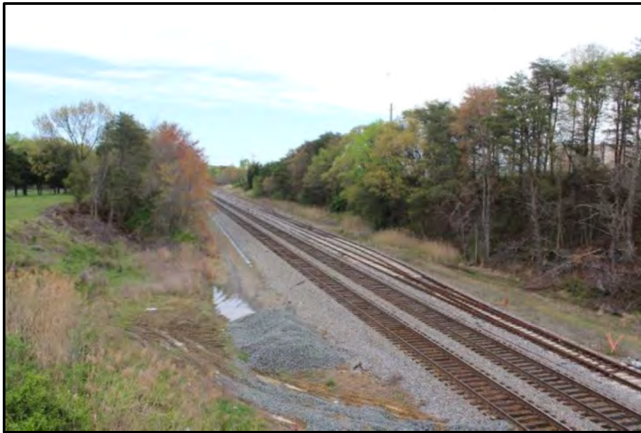
Figure 2 View of Richmond, Fredericksburg & Potomac Railroad (VDHR #076-0301), Richmond, Fredericksburg & Potomac Railroad Historic District (VDHR #500-0001), and the Cockpit Point Battlefield (VDHR #076-5842; Location 1) Looking North/Northeast.
