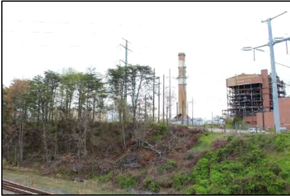
Figure 3 View from Richmond, Fredericksburg & Potomac Railroad (VDHR #076-0301), Richmond, Fredericksburg & Potomac Railroad Historic District (VDHR #500-0001), and the Cockpit Point Battlefield (VDHR #076-5842; Location 1) Looking Northeast towards Proposed Project Area.
