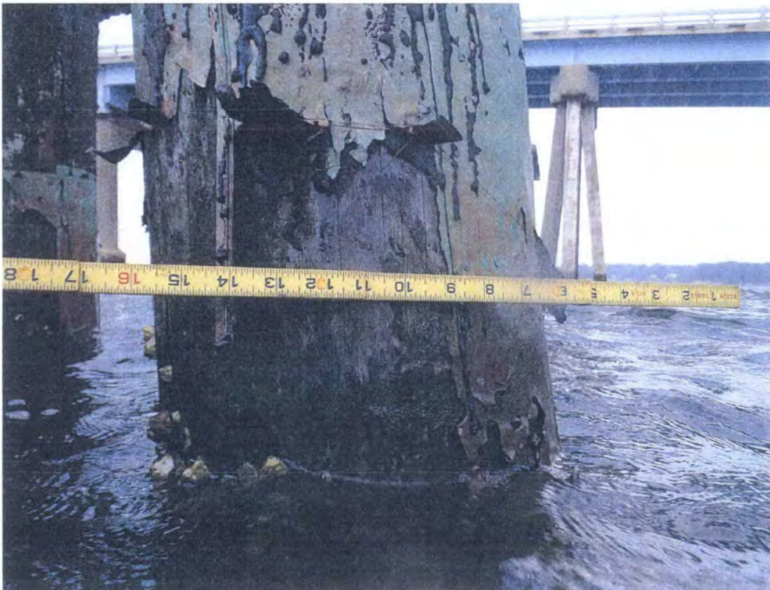
Missing Copper Sheathing (Typical)
