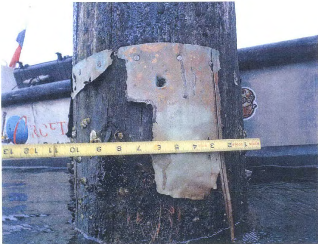
Missing Copper Sheathing (Typical)
