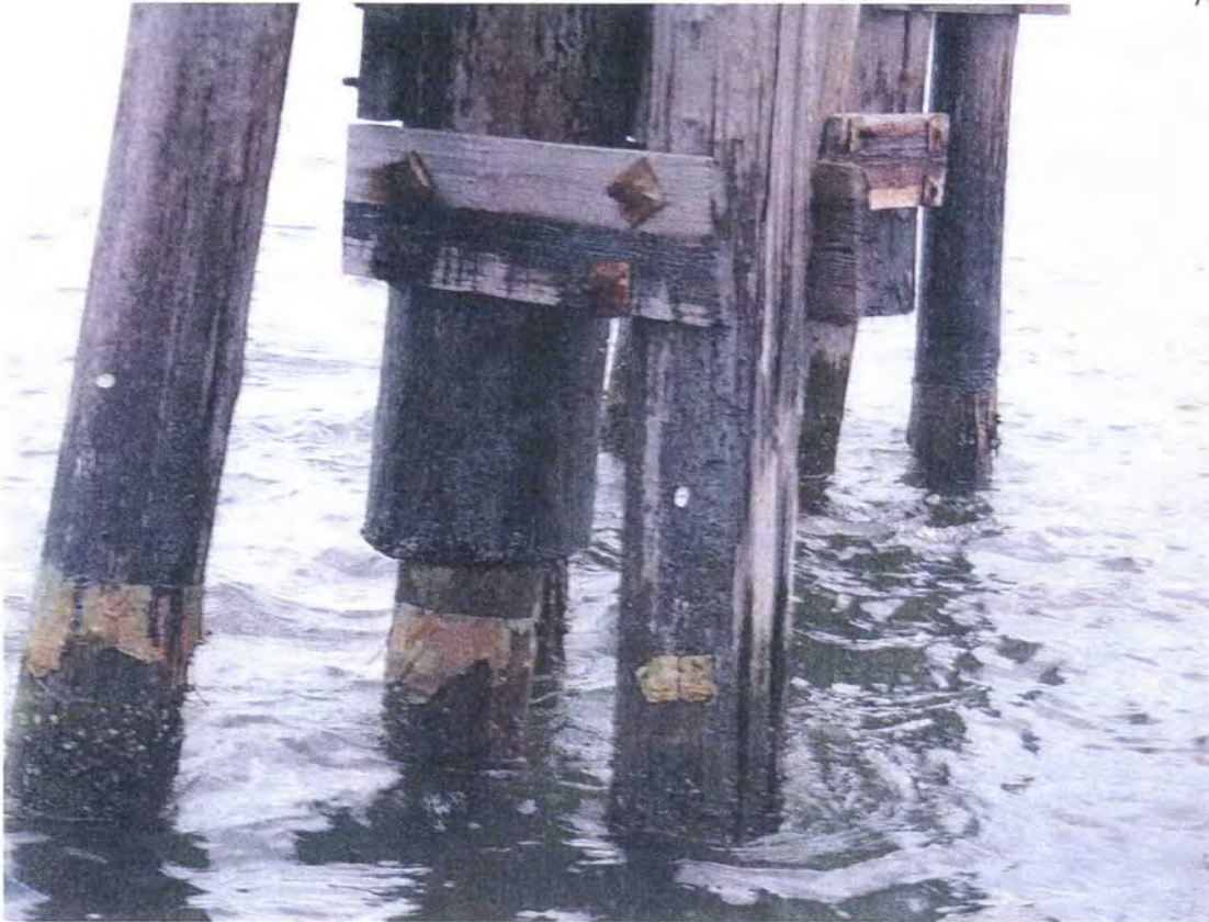
Missing Copper Sheathing (Typical)
