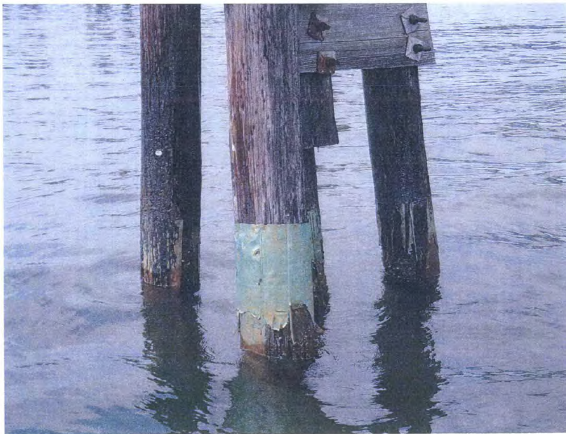
Missing Copper Sheathing (Typical)
