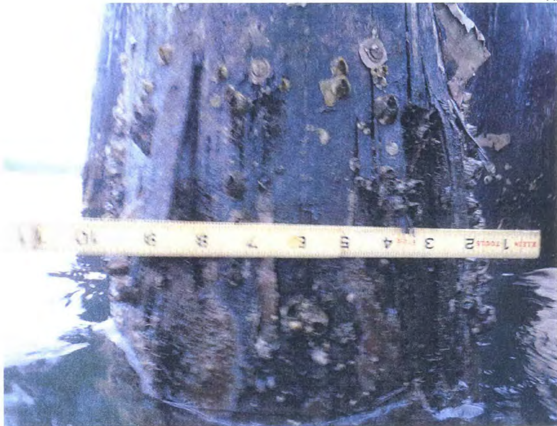
Waterline Deterioration
