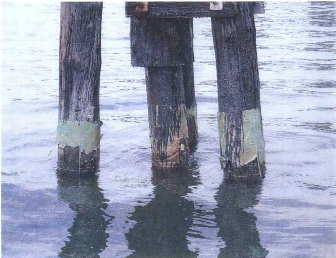
Missing Copper Sheathing (Typical)
