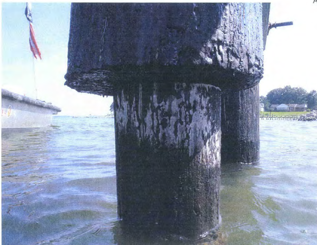
Waterline Condition (Typical)
