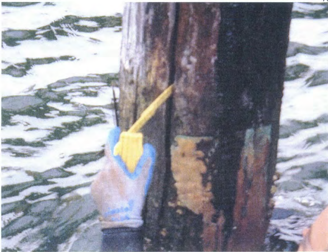
Waterline Damage
