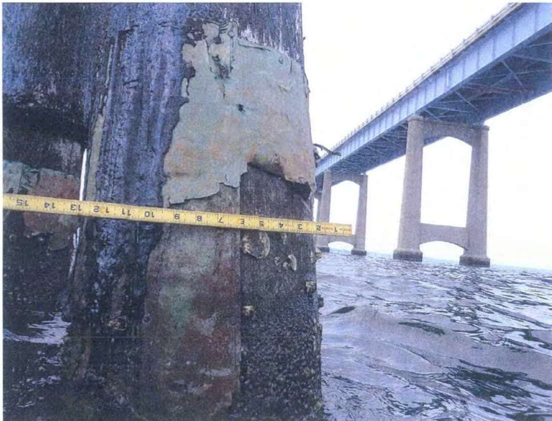
Missing Copper Sheathing (Typical)
