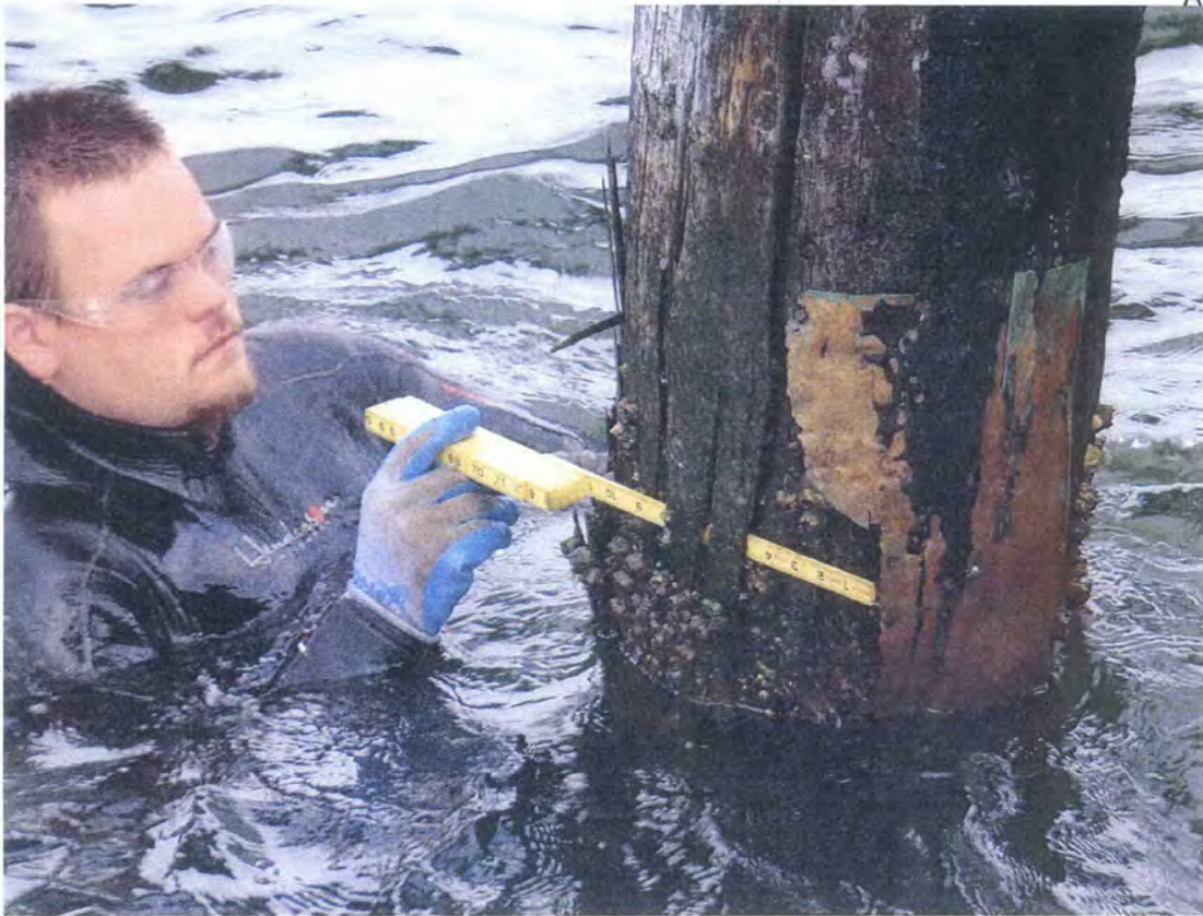
Waterline Damage
