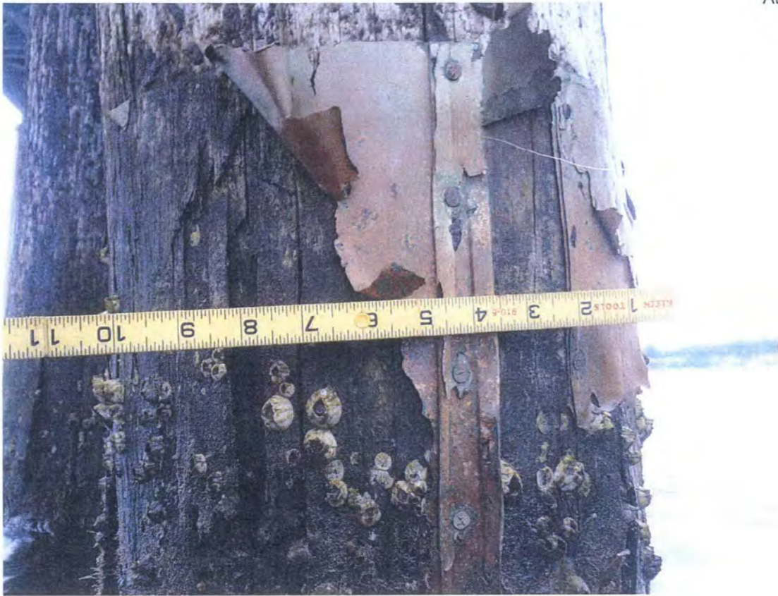
Waterline Deterioration
