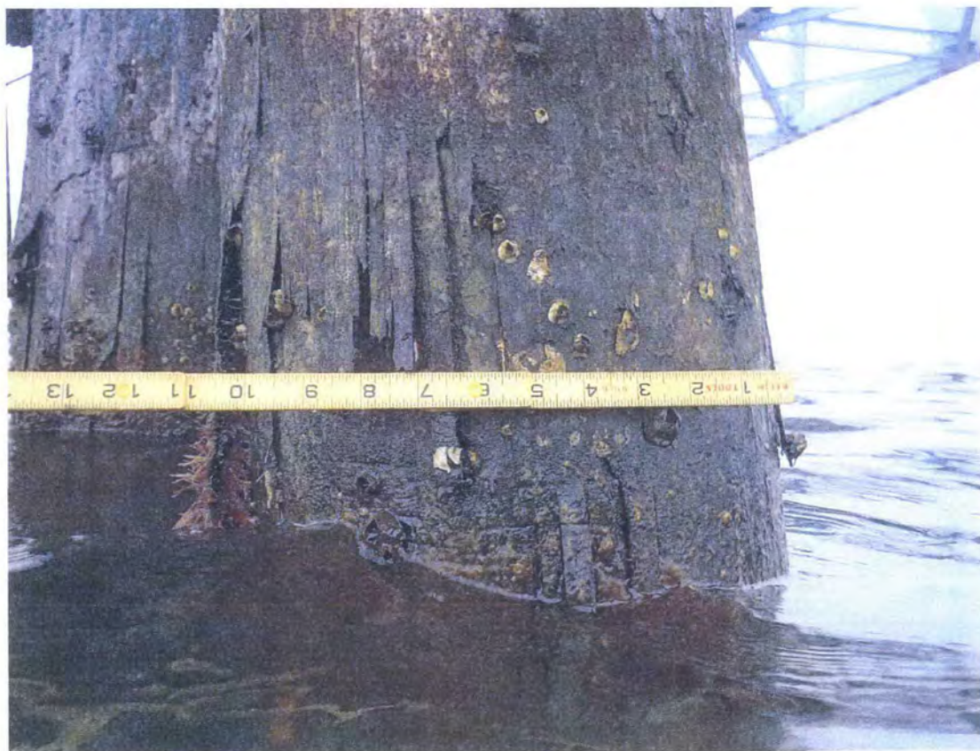
Waterline Deterioration
