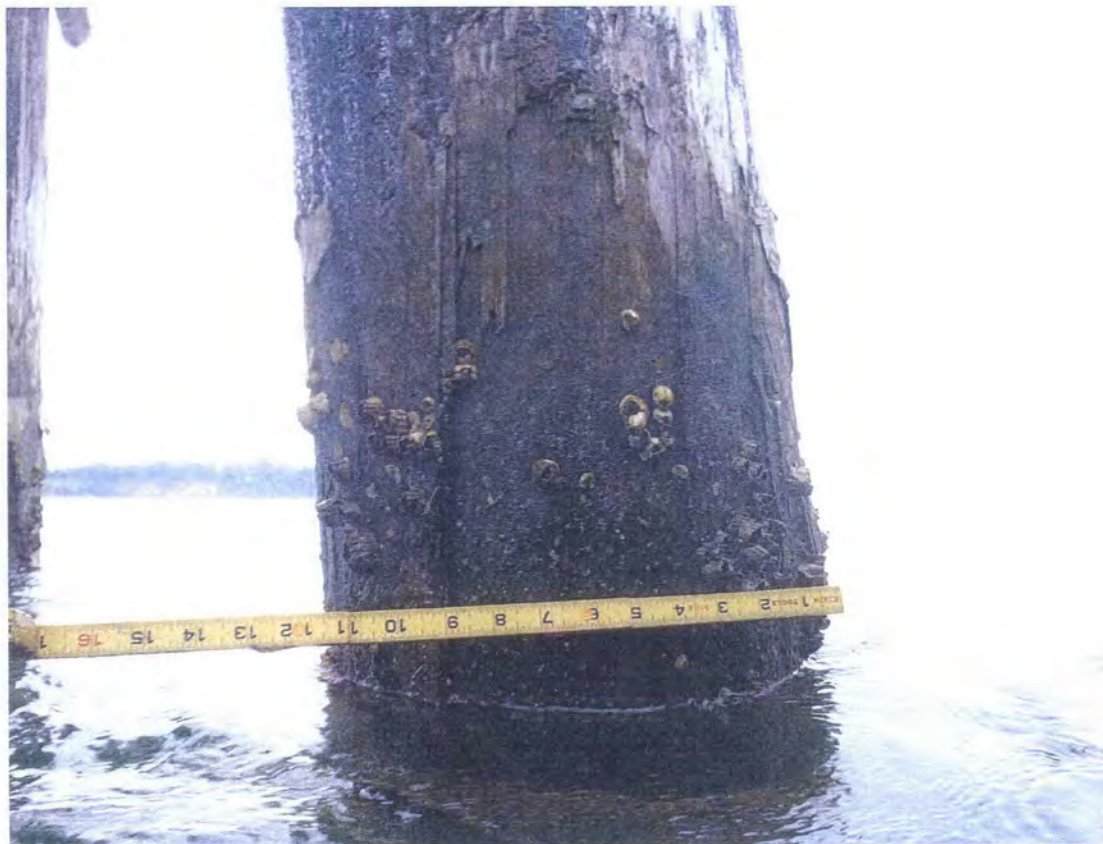
Waterline Deterioration
