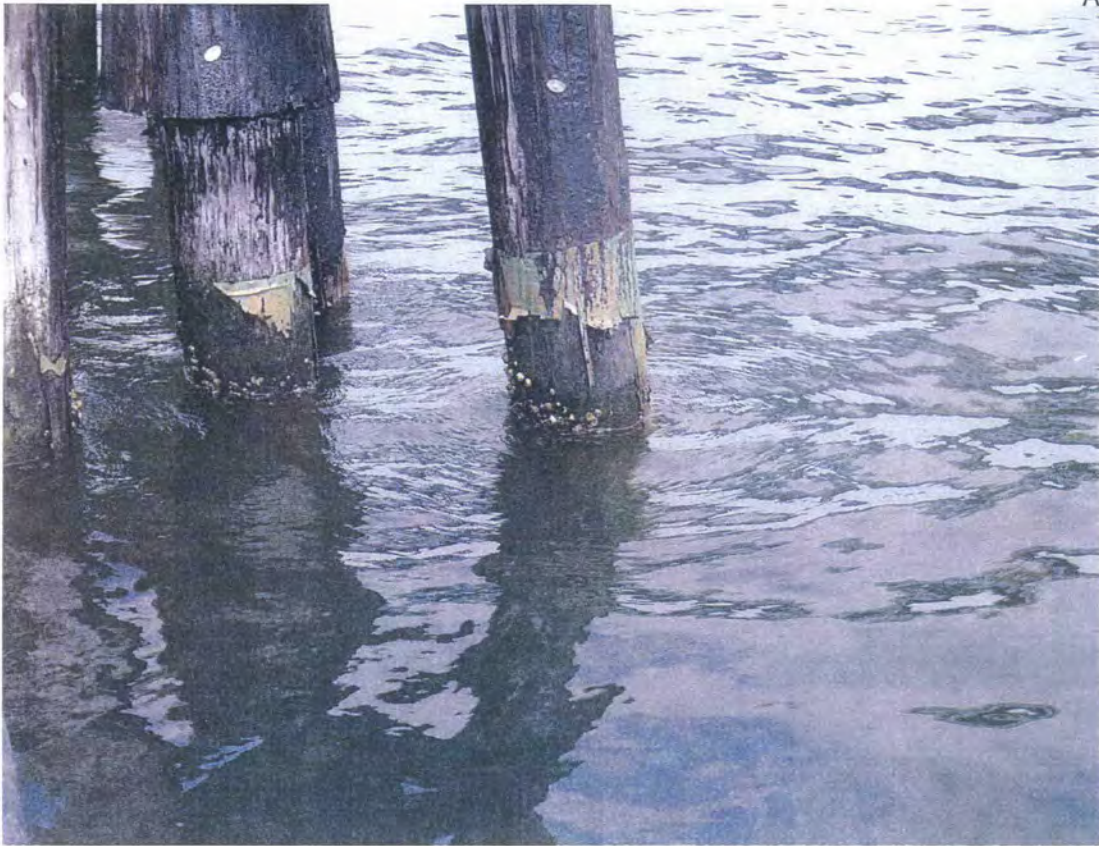
Missing Copper Sheathing (Typical)
