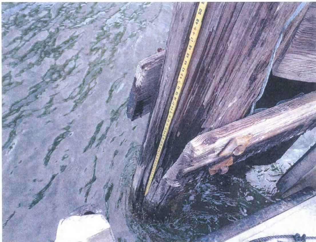
Waterline Damage
