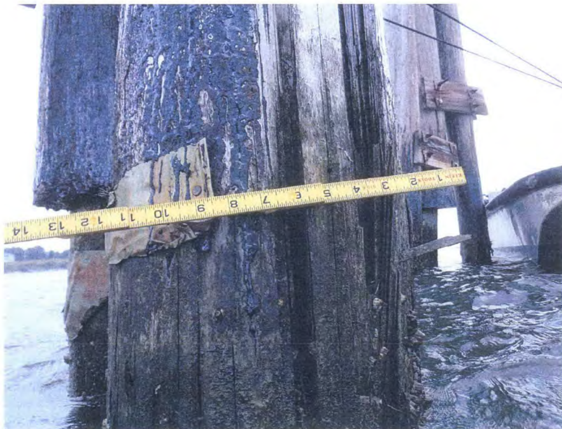
Waterline Damage
