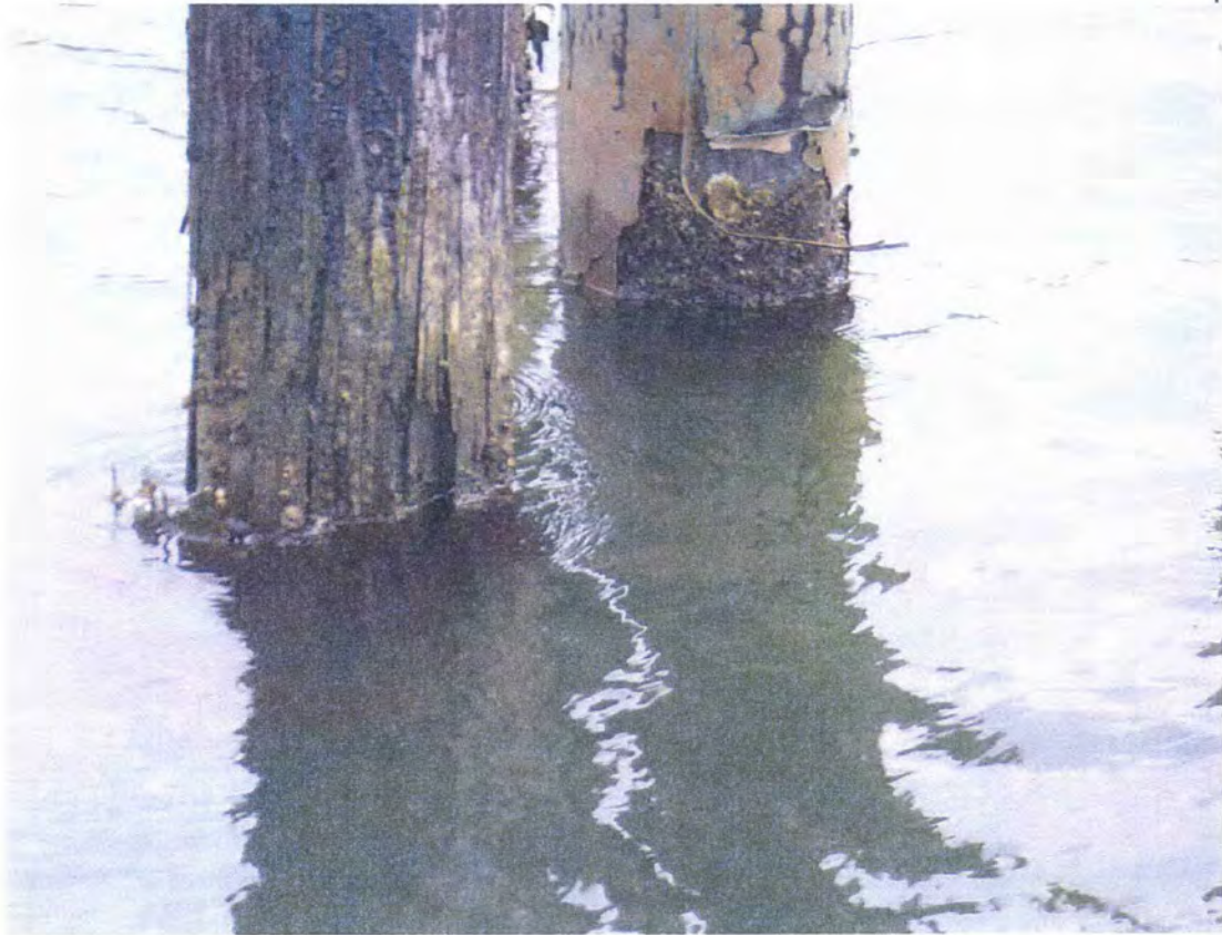
Waterline Deterioration (Typical)
