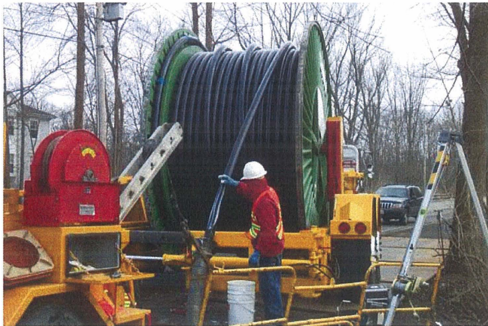
Land-based Cable Pulling – Reel Trailer Set Up
