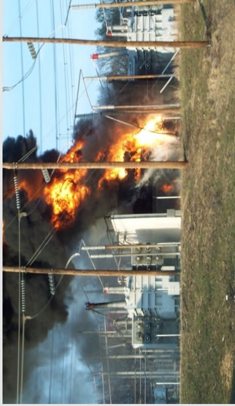
500 kV Transformer Failure in 2000
