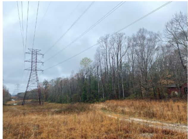
Existing weathering steel lattice towers north of the Chowan River, looking south. The 230 kV electric transmission line here shares structures with a distribution line to cross the wetlands and the river. Photo taken in March 2023.
