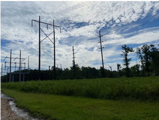
Existing transmission 230 kV H-frame and 115 kV monopole wooden structures by Tunis Substation in North Carolina. Photo taken in summer 2022.
