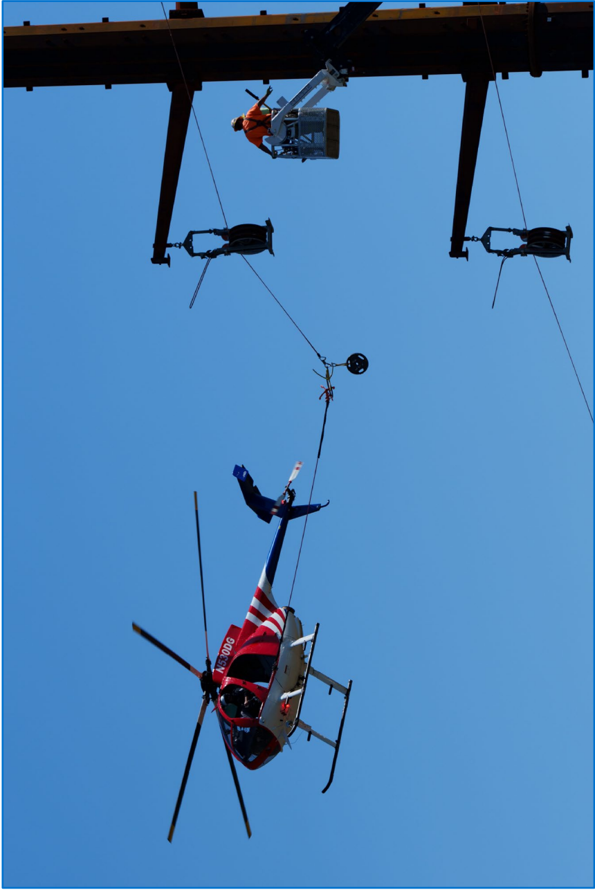
Helicopter helps install lines.
