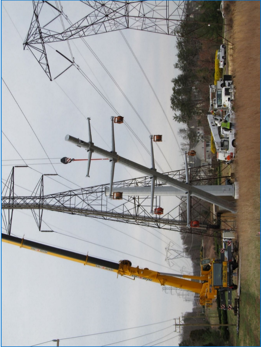
Cranes help assemble the pole pieces.
