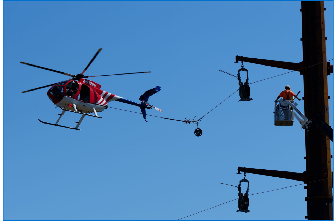
Helicopter helps install lines.
