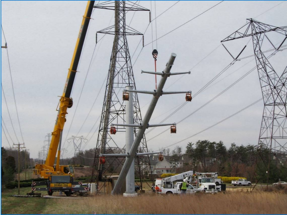
Cranes help assemble the pole pieces.
