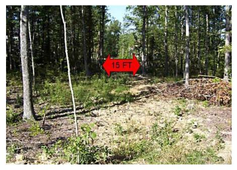
**Overhead 30' Right of Way -** The normal width of rights of way to be obtained for an overhead installation is thirty feet. Trees near the edge of the right of way need to be trimmed from the ground to the sky. This provides adequate clearance for the installation and maintenance of all overhead electric facilities. Additional easement may be required for down guys.
