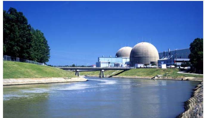
Surry Power Station; Surry County, VA.
