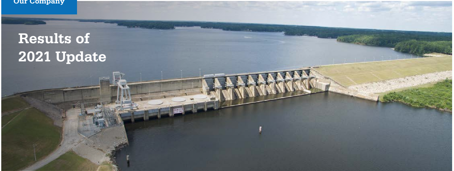
Gaston Hydro Station; Thelma, NC.
