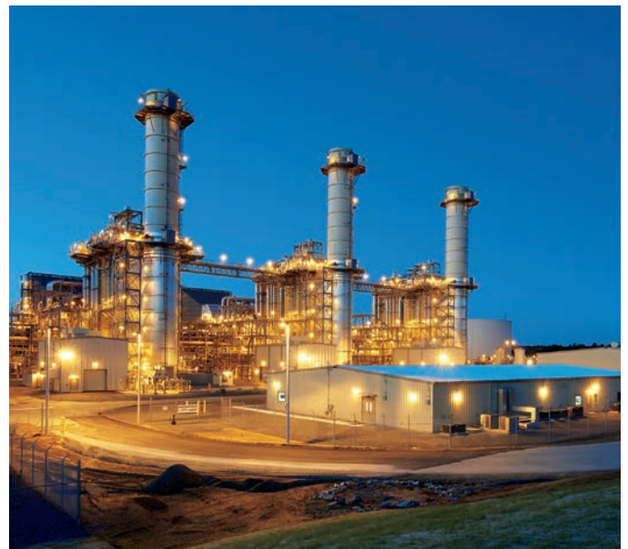
Brunswick Power Station.
