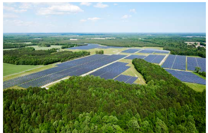
Southampton Solar Farm; Southampton, VA.
