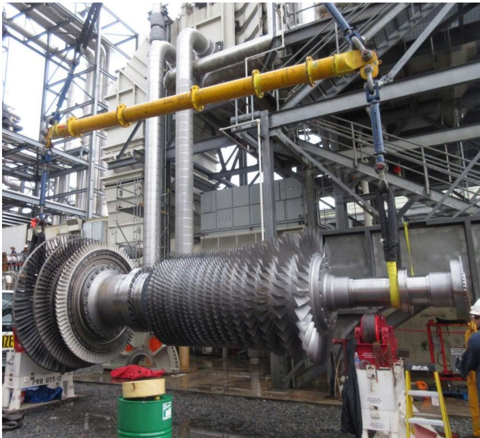
Figure 2: A Jasper Station Turbine Awaiting Installation after Maintenance and Upgrade
