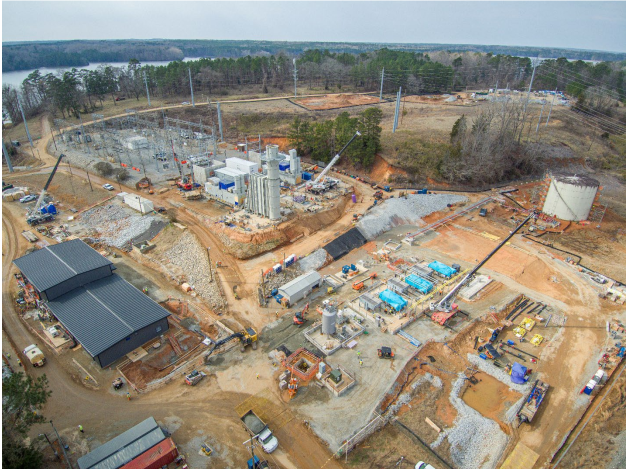
Figure 4: Construction Progress at Parr Station (As of February 5, 2025)
