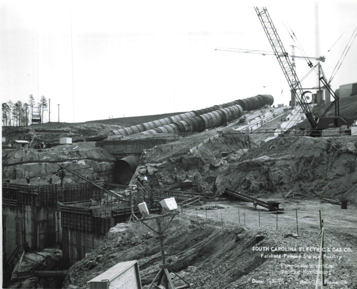
Construction of penstocks for Fairfield Pumped Storage
