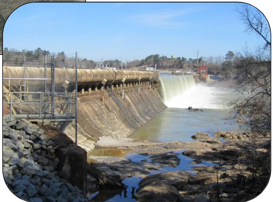
Parr Dam and Powerhouse (2016)
