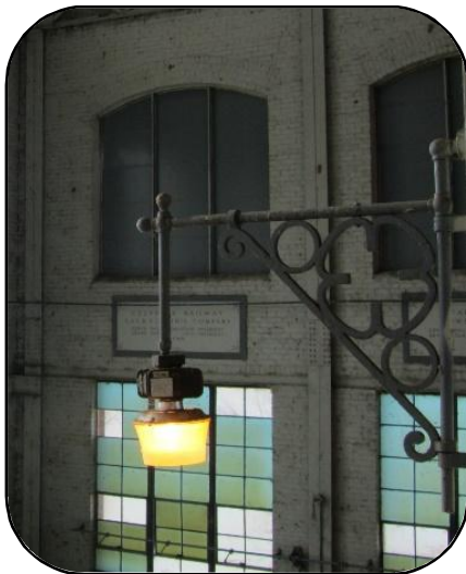
Lights within the Parr Powerhouse
