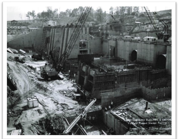
Fairfield Powerhouse construction (1976)
