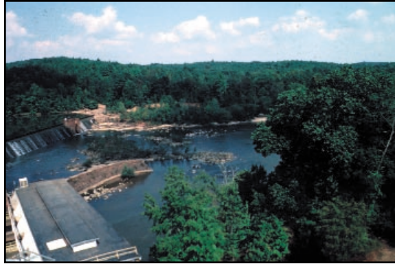
The Neal Shoals Hydroelectric Facility.
