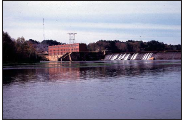
The Stevens Creek Hydroelectric Facility.
