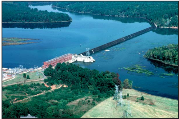
Aerial View of the Stevens Creek Hydroelectric Facility.
