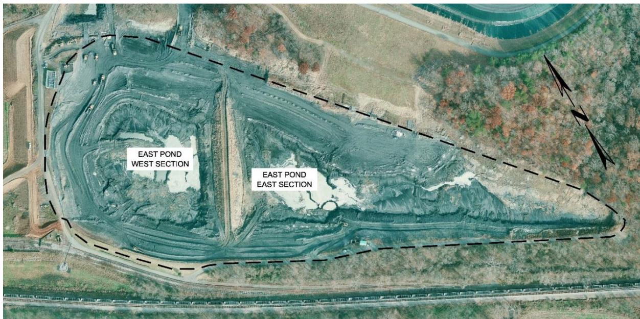
Figure 1 - December 2017 East Ash Pond Aerial Photo
