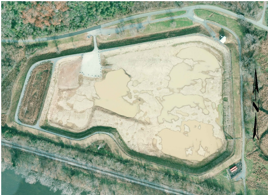
Figure 1 - December 2017 West Ash Pond Aerial Photo
