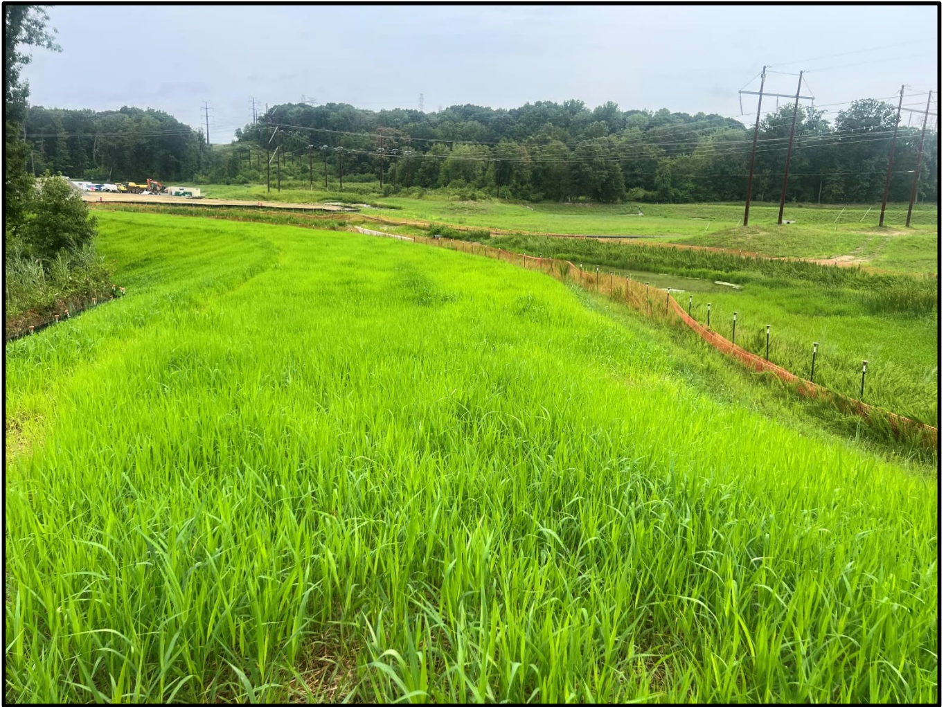
Photo 4 - Ponds ABC Repairs Looking North towards Sections C-C' and B-B'
