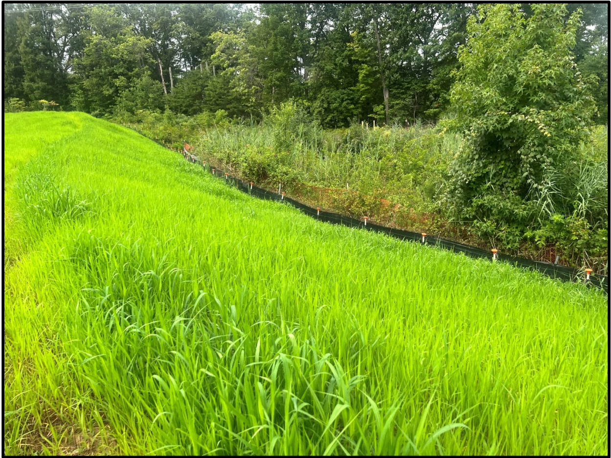
Photo 3 - Ponds ABC Repairs Looking South-Southwest at Section C-C'
