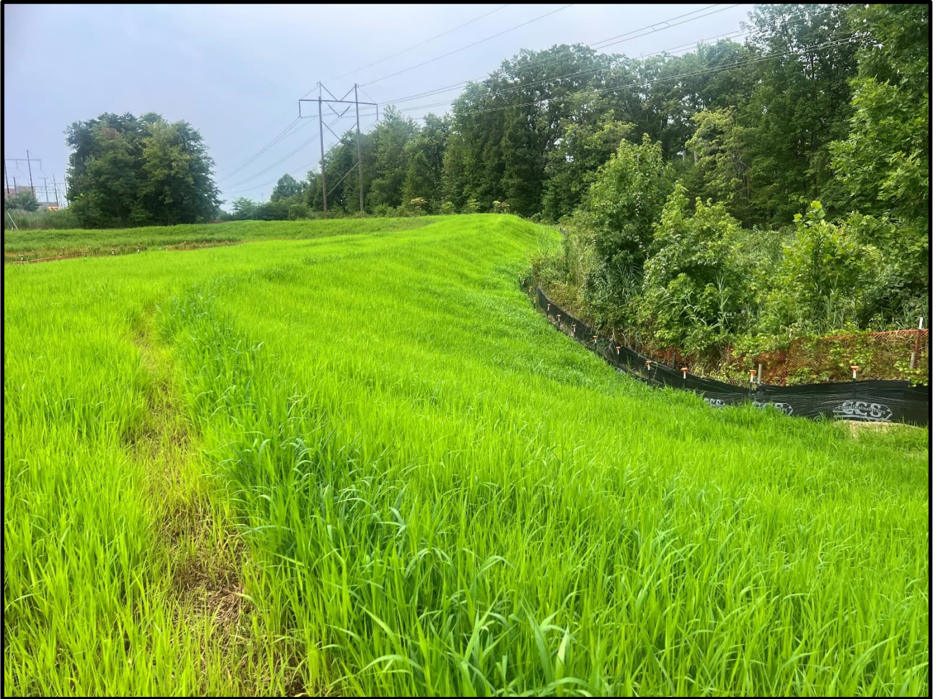
Photo 2 - Ponds ABC Repairs Looking South adjacent to Section C-C'
