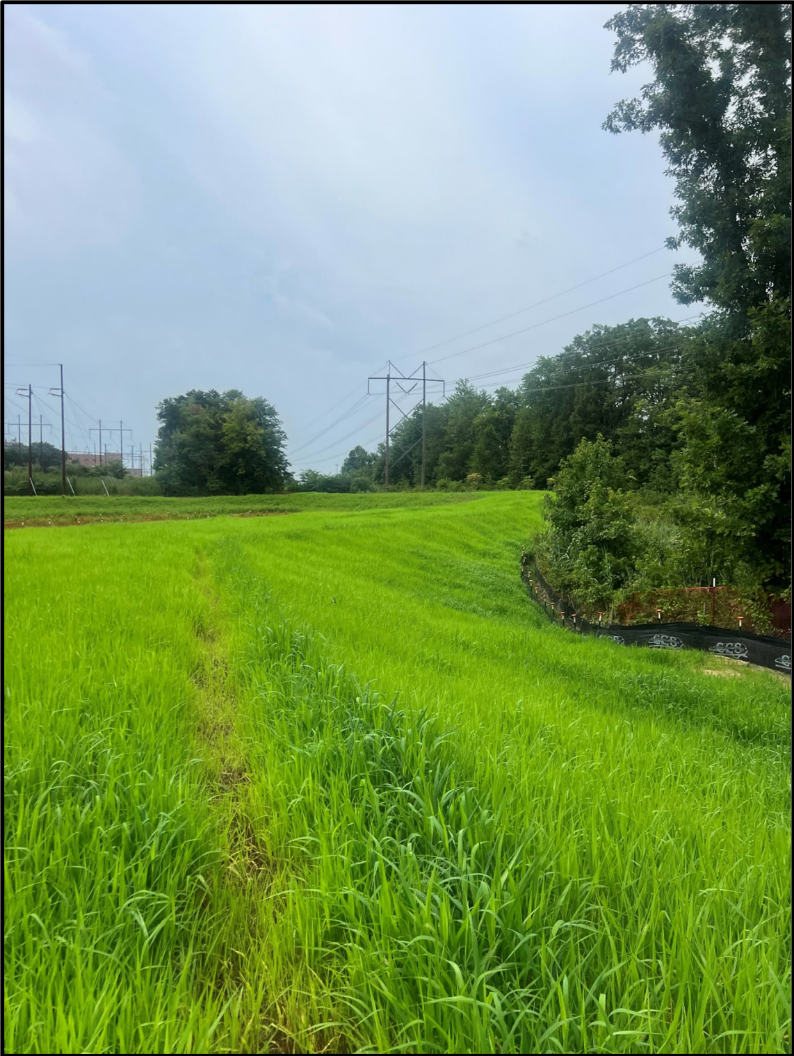
Photo 1 - Ponds ABC Repairs Looking South towards Sections B-B' and C-C'
