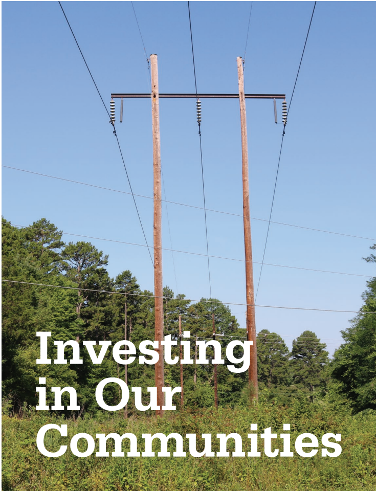
Dominion Energy image. Not project specific.
