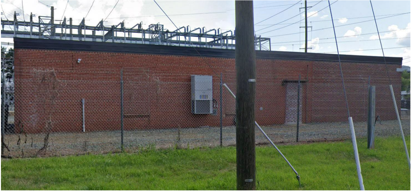
Existing Charlottesville Substation Control Enclosure View from Smith Street
