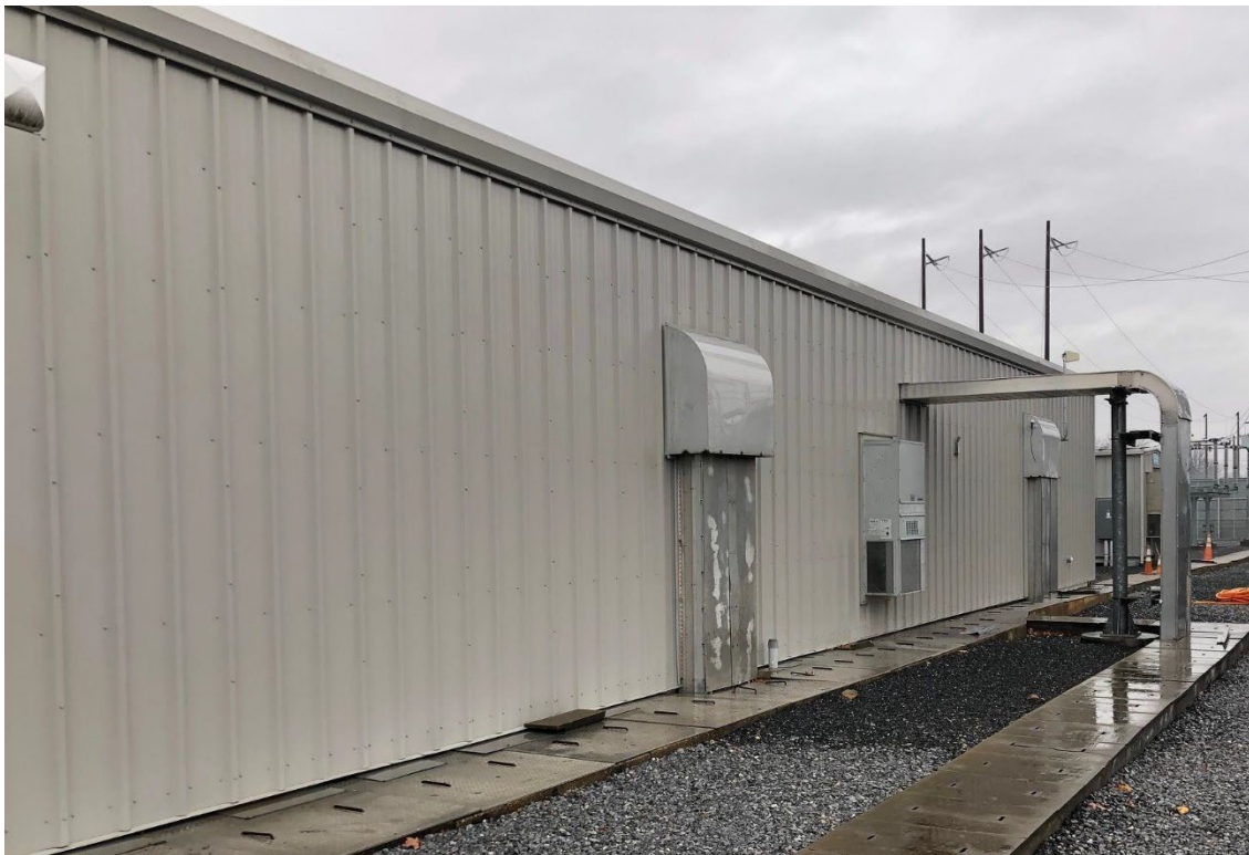
Typical Encapsulated Control Enclosure (in progress)
