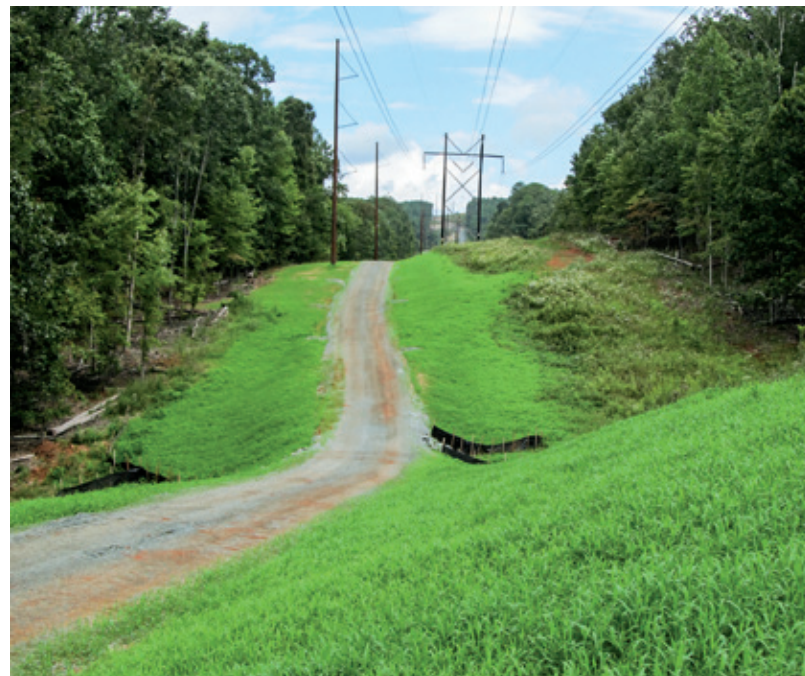
Crews install erosion control blankets (above) to protect the ground while new grass takes root (below).
