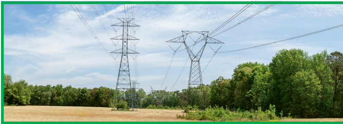
Existing Corridor 1B – lattice tower (left) will be reconducted. New monopoles will be installed to the left of these structures. Visit the Backyard Application on the project website to view visuals of the proposed monopole structures.
