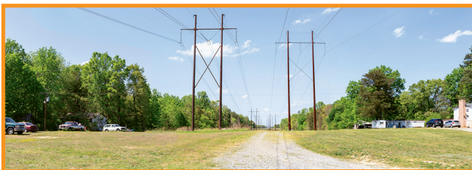
Existing Corridor 3: H-Frame structures (left) will be replaced with new monopole structures. No replacement of structures on the right.
