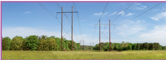
Existing Corridor 2: H-Frame structures (left) will be replaced with new monopole structures. No replacement of structures on the right.
