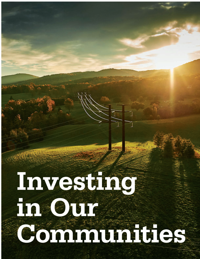
Dominion Energy image. Not project specific.
