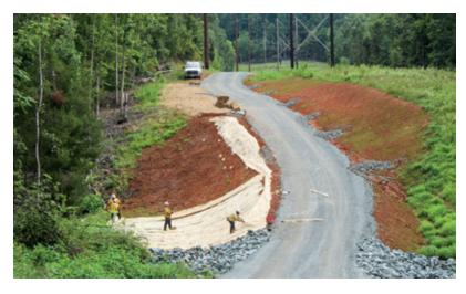
Crews install erosion control blankets (above) to protect the ground while new grass takes root (below).
