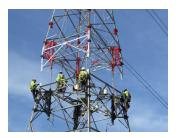
Qualified technicians install the self-contained, hydraulically driven "crane" in the structure. This slowly and safely lifts the structure, allowing permanent supports to be installed without interrupting power flow.
