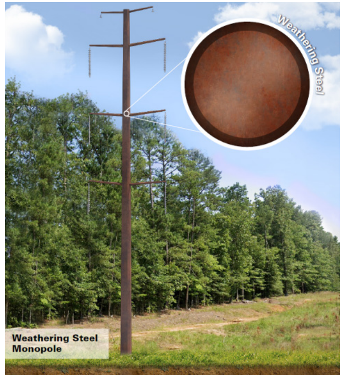
Example of double-circuit monopole overhead structure
