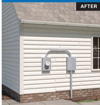
A "junction box" adapter can be installed utilizing entrance cable to connect the meter base to the adapter.
