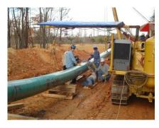
Welding steel pipe together. Welds are then radiographically inspected (xrayed) to ensure pipe joints have been welded in accordance with project specifications.
