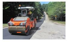
The final phase, cleanup and restoration, involves removing construction material, installing a final layer of asphalt and restoring the area.
