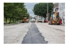
Backfilling trench and a temporary asphalt patch is added, while ensuring pipeline is protected from rocks or debris.
