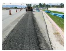
Digging trench to specified depth (typically 4') for pipe placement.
