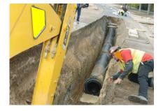
Lowering pipe into trench. Trench is cleared of rocks and debris.
