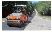
The final phase, cleanup and restoration, involves removing construction material, installing a final layer of asphalt and restoring the area.
