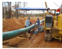
Welding steel pipe together. Welds are then radiographically inspected (x-rayed) to assure pipe joints have been welded in accordance with project specifications.
