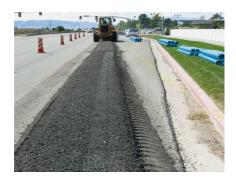
Digging trench to specified depth (4' typical) for pipe placement.
