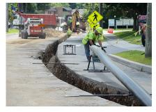
"Installing" pipeline section into the trench.
