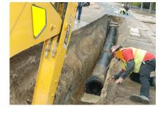
Pipe is lowered into trench. Trench is clear of rocks and debris.
