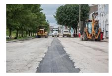
Trench is backfilled and a temporary asphalt patch is added while ensuring pipeline is protected from rocks or debris.
