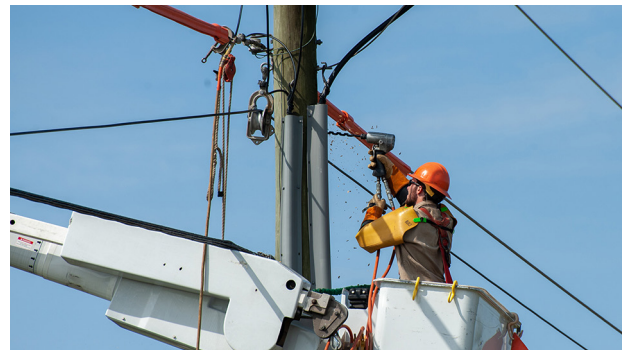
An authorized Dominion Energy contractor installs permanent fiber attachment hardware.
