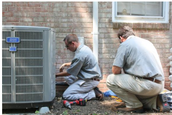
Installing the AC Cycling Switch
