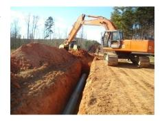
The trench is then **backfilled**. When soil conditions are not suitable to be directly placed on the pipe, specialized equipment designed to pad the pipe and protect it from sharp rocks and abrasion is utilized.
