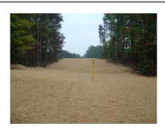
The final phase of the construction is **cleanup and restoration** of the right-of-way. This involves replacing topsoil, replanting the right-of way, removing construction material, and restoring the area, as closely as possible, to its original pre-construction condition.
