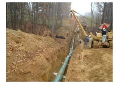
The pipe joints are cleaned and coated and the ditch bottom is cleared of rocks and debris or padded with soft dirt and the pipe is **lowered-in** to the ditch by sideboom tractors using belts or cradles in a carefully coordinated action. The ends of the pipe segments are then welded together to form one continuous pipeline.
