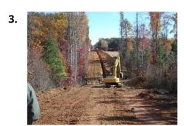
Next, the mechanical excavation of a trench, dug to a specified depth for pipe placement, is done by the **trenching** crew. Occasionally, rock drilling and blasting is required to break rock in a controlled manner.
