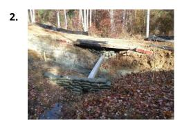
All waterway crossings are flagged prior to clearing to indicate the minimal disturbance zone where equipment and work activities are restricted until the waterway crossing takes place. Access over watercourses is facilitated by using portable bridges installed to span the waterway.
