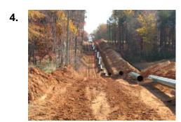
After the pipe is delivered to the right-of-way, the contractor **"strings"** segments of steel pipe by laying the pipe joints on wooden skids adjacent to the trench.
