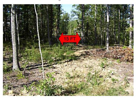
**Overhead 30' Right of Way -** The normal width of rights of way to be obtained for an overhead installation is thirty feet. Trees near the edge of the right of way need to be trimmed from the ground to the sky. This provides adequate clearance for the installation and maintenance of all overhead electric facilities. Additional easement may be required for down guys.
